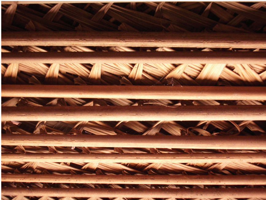
Foto 7: Daun bertam yang disisip menjadi lelangit. Photo 7: Bertam leaves inserted to become the ceiling. (Sumber : Jabatan Warisan Negara, 2010) (Source: Department of National Heritage, 2010)
