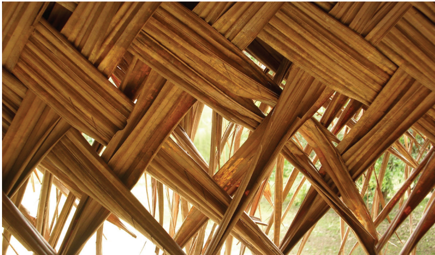
Foto 6: Daun bertam dijadikan atap. Photo 6: Bertam leaves made into roofing. (Sumber : Jabatan Warisan Negara, 2010) (Source: Department of National Heritage, 2010)
